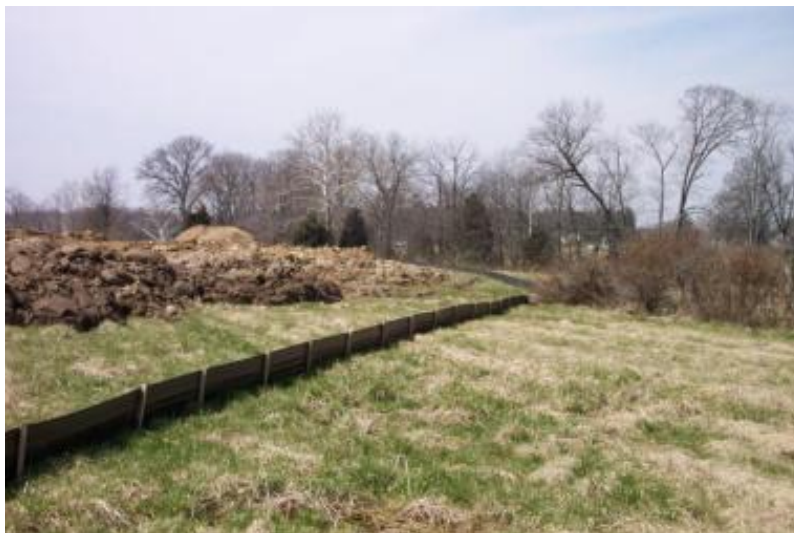
Figure 5 – Typical silt fence
